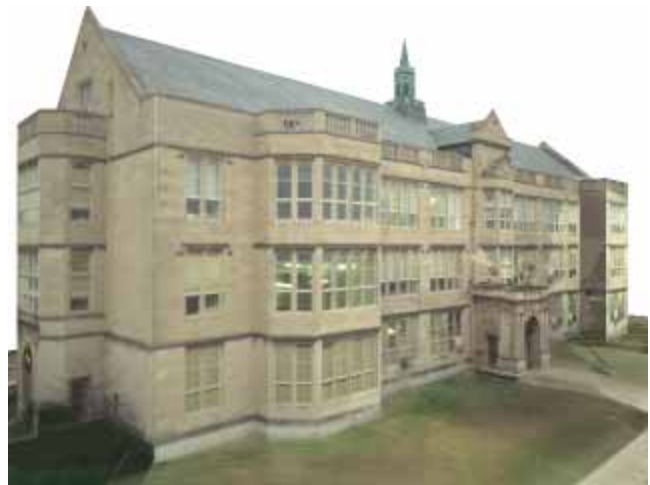
Figure 9: A synthetic view of University High School. This is a frame from an animation of flying around the entire building.
